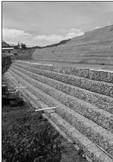
**Figure 3:** Application of a reinforced soil slope with polymeric and metallic reinforcement for an airport runway construction (courtesy of PT. Maccaferri Indonesia).
