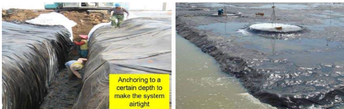
Figure 10. Anchoring geomembrane along the perimeter of target improve area
