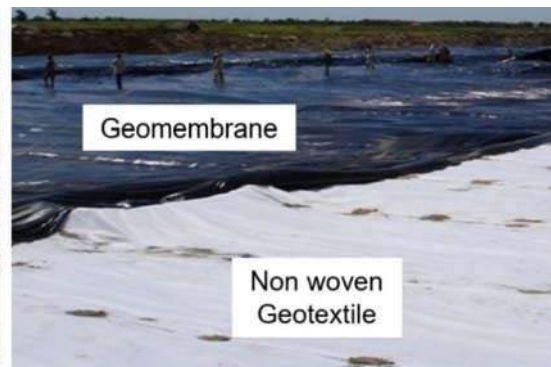
Figure 9. Geotextile & geomembrane installation
