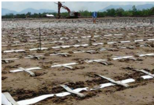
Figure 8. PVDs & horizontal drains installation
