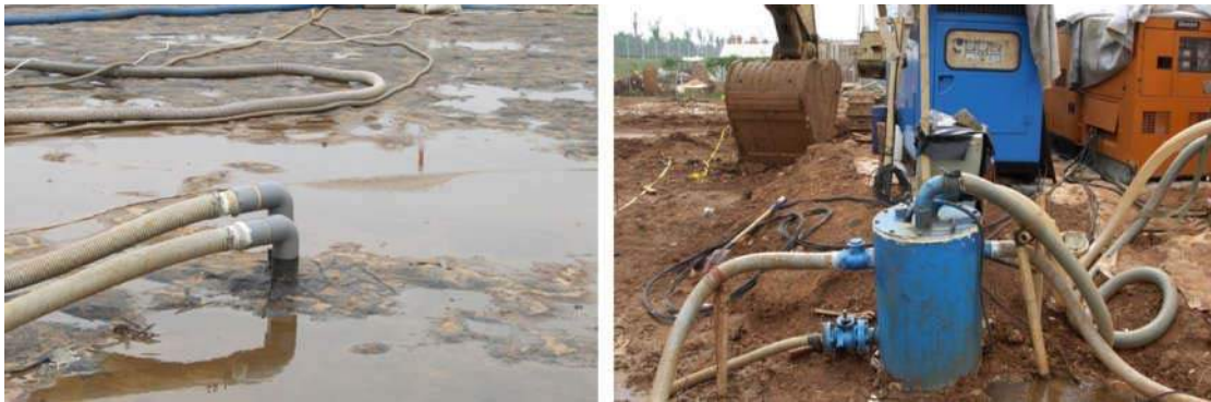
Figure 11. Connect the piping system to the vacuum pump
